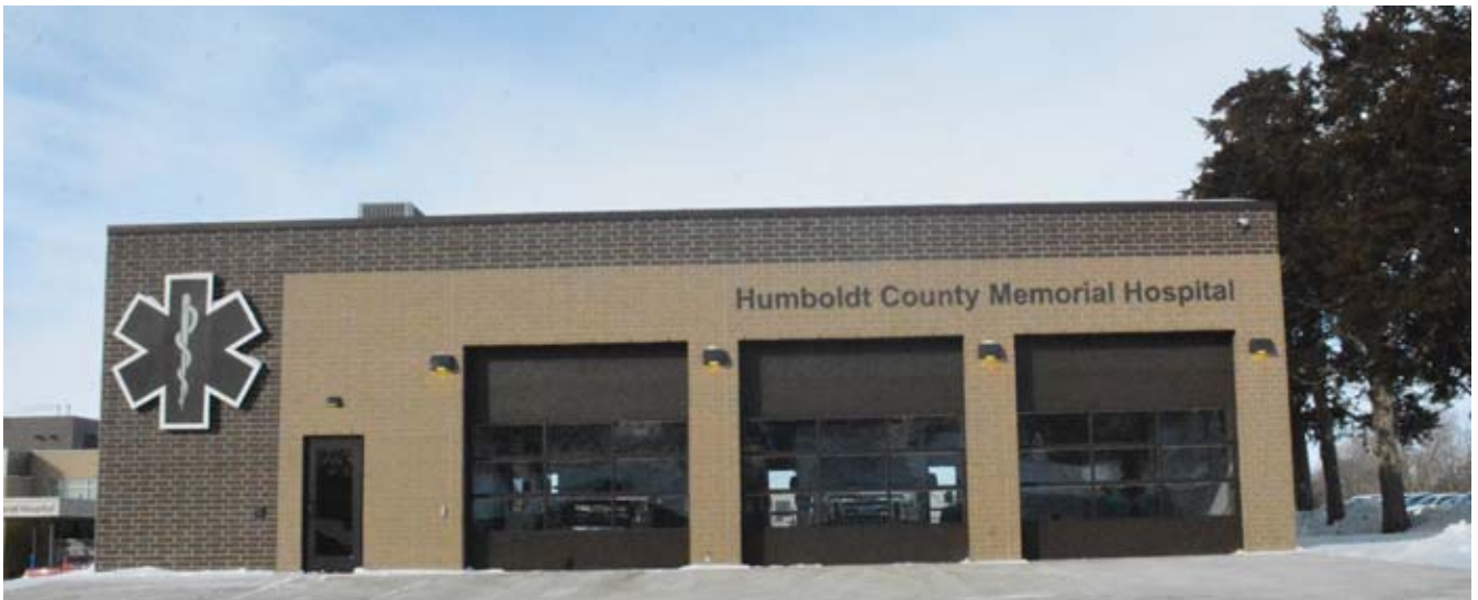
HCMH finished their new ambulance garage in the summer of 2021 in response to the COVID pandemic. The garage was used as a drive-through location for testing as well as a dedicated spot for the ambulance service
